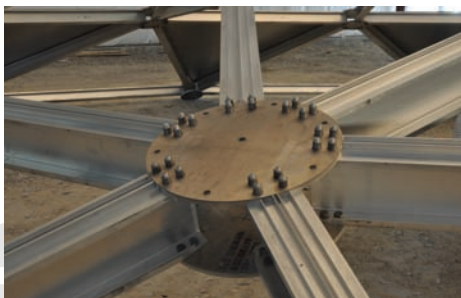
Node detail utilizes proprietary extrusion design.
