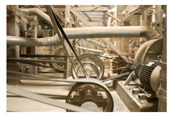
Another important component in a ventilation system is the ductwork. If the particulate does not have an opportunity to reach the baghouse, the dust collector will not be able to perform its function. Standard practices suggest a minimum airstream velocity within any duct of 3500 feet per minute (fpm), and between 4000 and 4500 fpm for heavier dusts, such as sand. If the dust travels at lower than adequate velocities, it will tend to settle and accumulate in the ducts, choking the system.
