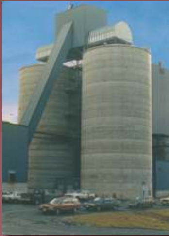
Model 698 Systems with concrete silos
