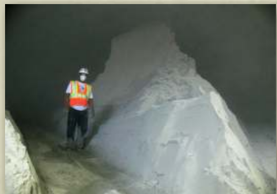
Pie-shaped piles of hard-packed material remain after operation air-gravity conveyors.
