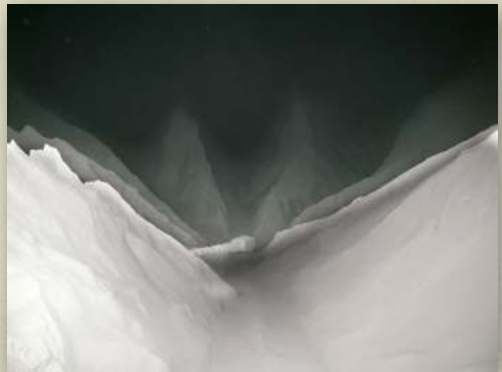
Initial reclamation via air-gravity conveyors reclaims a large percentage of the stored material, and allows the screw to start under minimal load.
