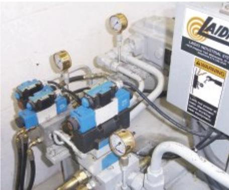
The two-speed hydraulic reclaim drive incorporates an advanced torque-sensing control to auto-shift from low-rpm/high-torque for heavy loads to high-rpm/low-torque for lighter loads.
