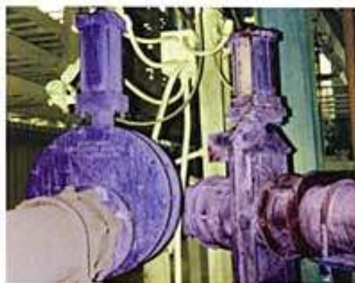
BMV replaces segregation line knife gate valves in flangeless piping.
