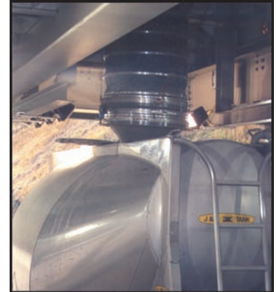
Trucks are loaded dust free at rates to 1000 TPH.
