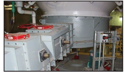
Aerated bin bottom with side discharge and flow control valves.
