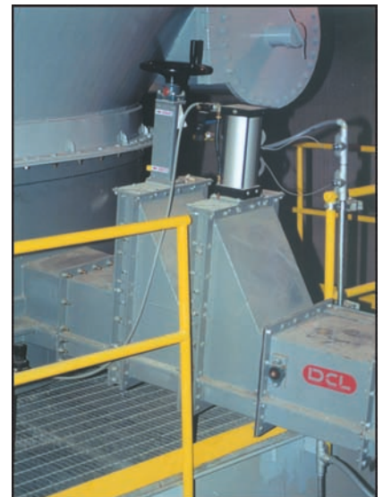
Vertical manual and pneumatic slide gate valve.
