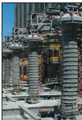
Ship loading spouts utilizing compact filter modules
