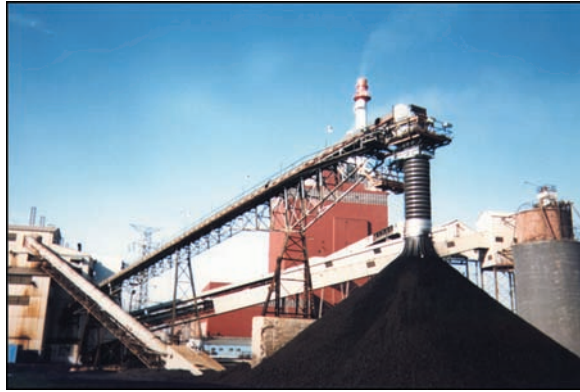
Dust free coal stockpiling.
