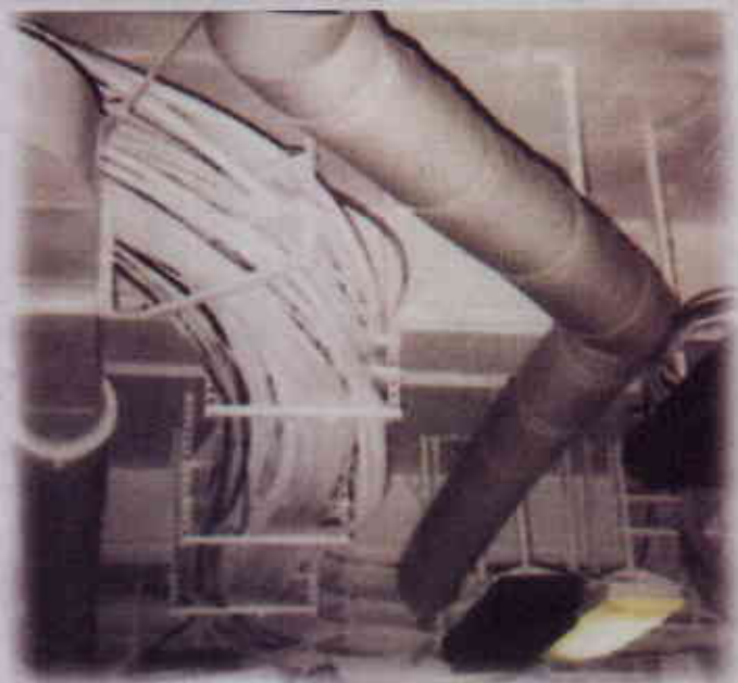
Tex-Duct can be configured to zig-zag left and right around any obstruction.
