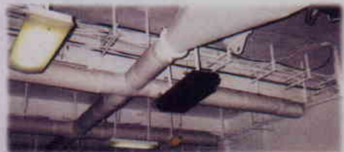
Tex-Duct consumes less space than the original steel ducting, reducing weight and saving precious space. Standard zipper construction allows for future modifications.
