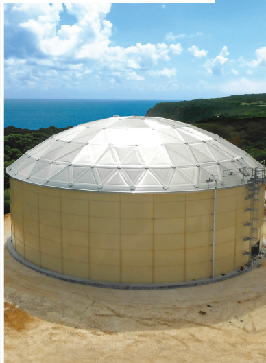
RTP potable water storage
