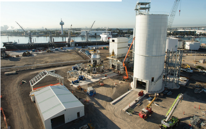
RTP dry bulk silo under construction
