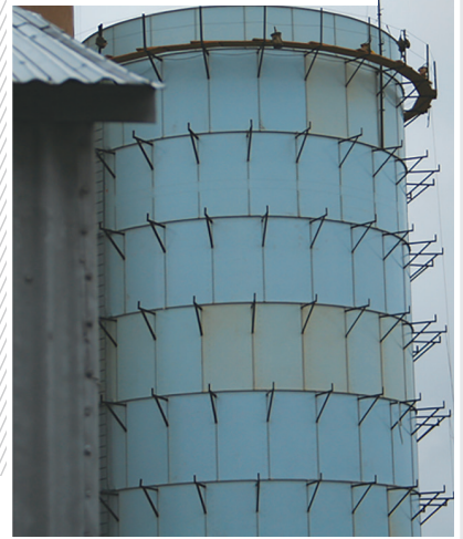
API 12B flanged panel tank - scaffold built
